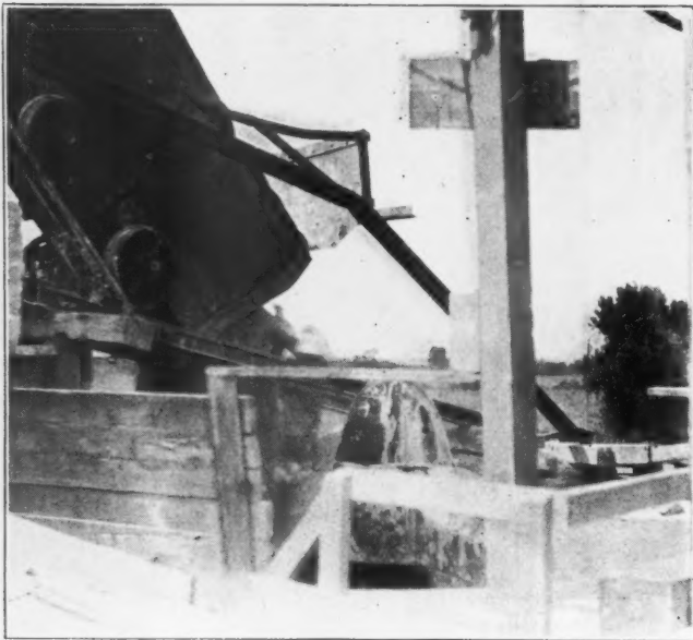
Discharging to Crusher
